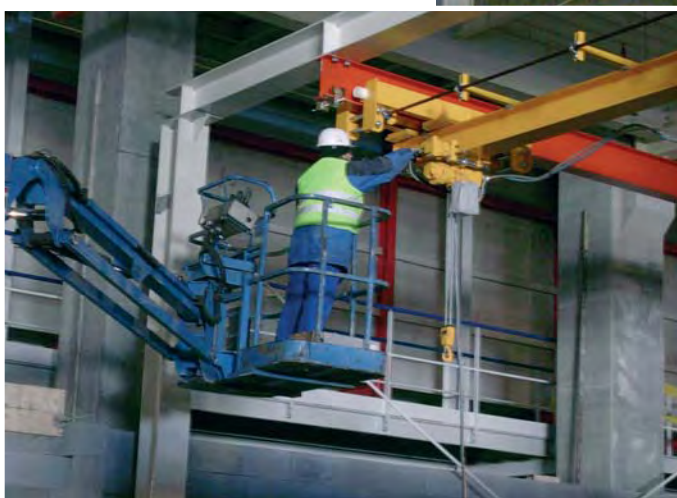
crane installation
