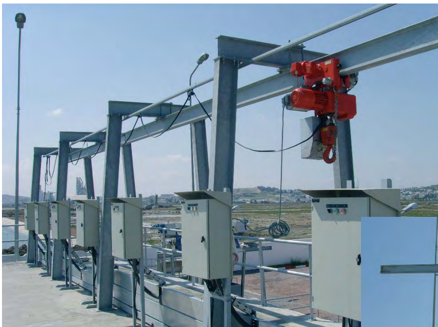
Electric Chain Hoist with electric trolley Type 66/04 AKE capacity: 5 t installed in a sewage plant in Tunisia
